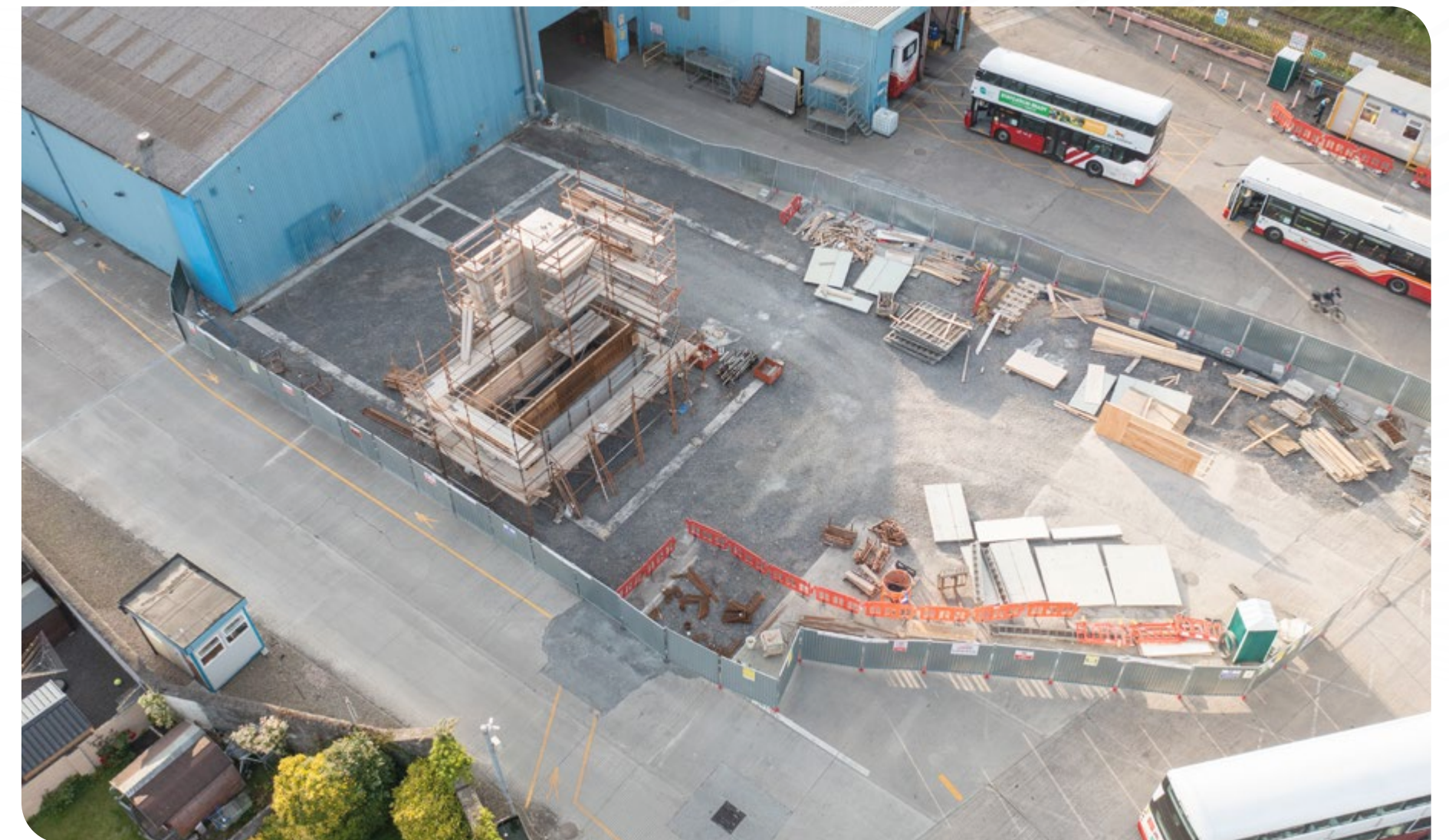
Works commencing at Roxboro, Limerick.
